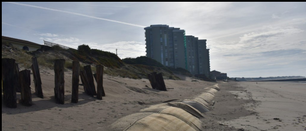
Sleeper corridor (tuboflex). Sleeves of sand with 2.40 meters.
